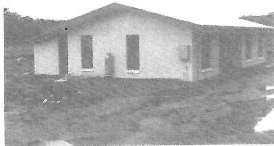
Caretaker's residence opposite Sports Centre.
